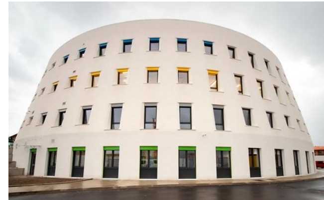
Central Storage of Museum of Applied Art in Prague, Praha -Stodůlky
